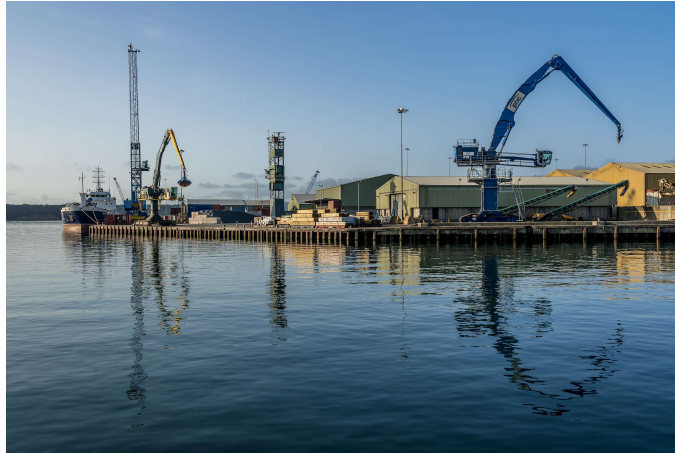
WG 233 "Inspection, maintenance and repair of waterfront facilities"
